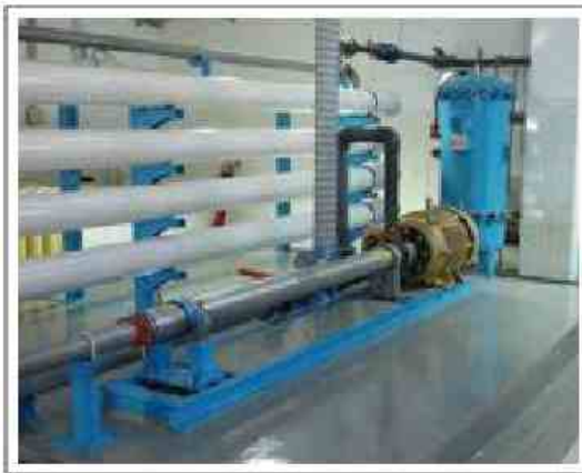
MSS with FEDCO baseplate
